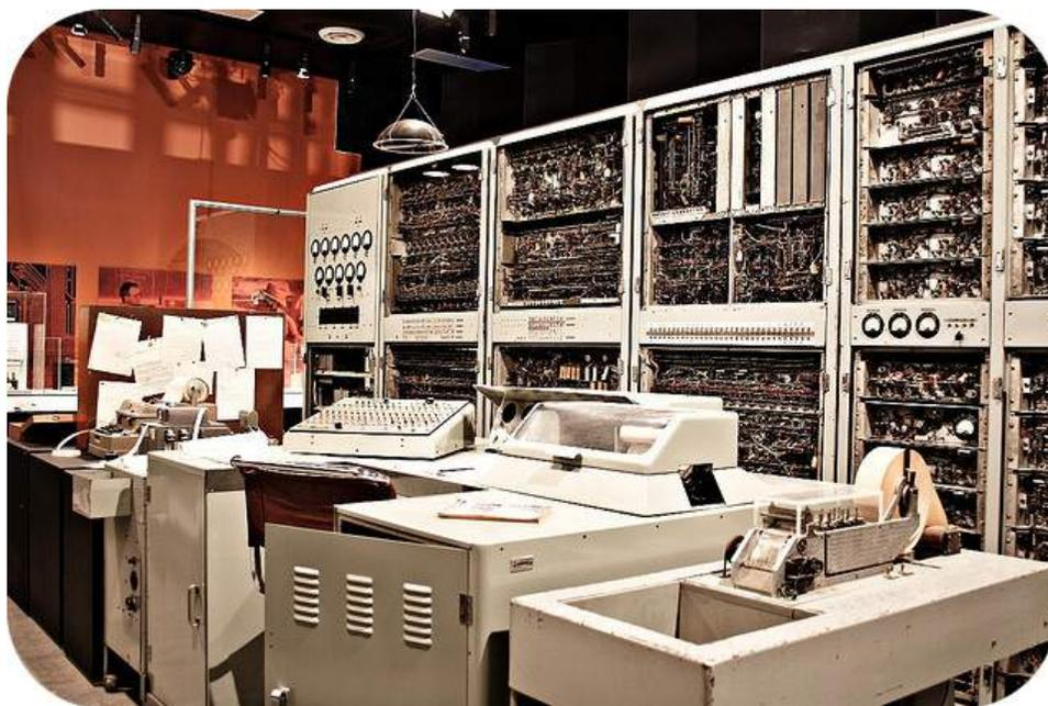
Scientists use computers to aid with all the mathematics needed to do science. Computers take and store measurement readings and do hours of mathematical calculations. The image is of the CSIRAC (Council for Scientific and Industrial Research Automatic Computer), Australia's first digital computer, first run in November 1949. This room-filling computer was able to do less than the personal computers of today.
