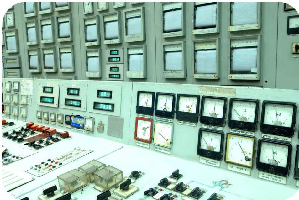
This photo is of the interior of the control room for a nuclear power plant. Many of the meters are reading information about the water temperature and the nuclear reaction that is occurring, but the majority of the meters are reading data about the electric energy being generated.
