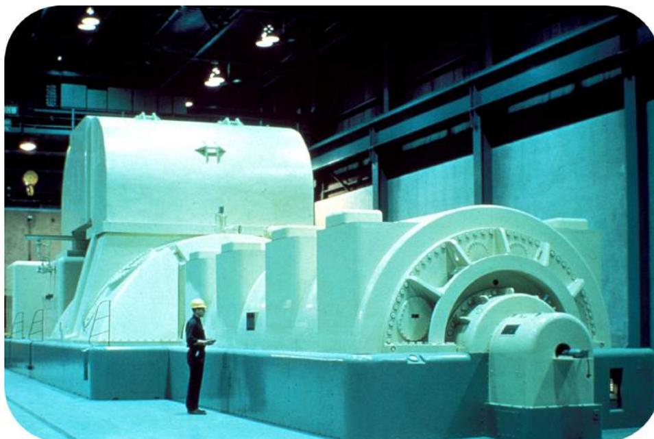
Electrical generators convert mechanical energy into electrical energy. Every electrical generator needs some method for spinning the coil inside the magnetic field. Hydroelectric generators use water pressure to spin the coil while windmills, of course, use the wind to spin the coil. The image here is a combination of steam turbine and generator. The steam can be produced by burning coal or diesel fuel or by a nuclear reaction and the steam then turns the coil and generates electricity.
