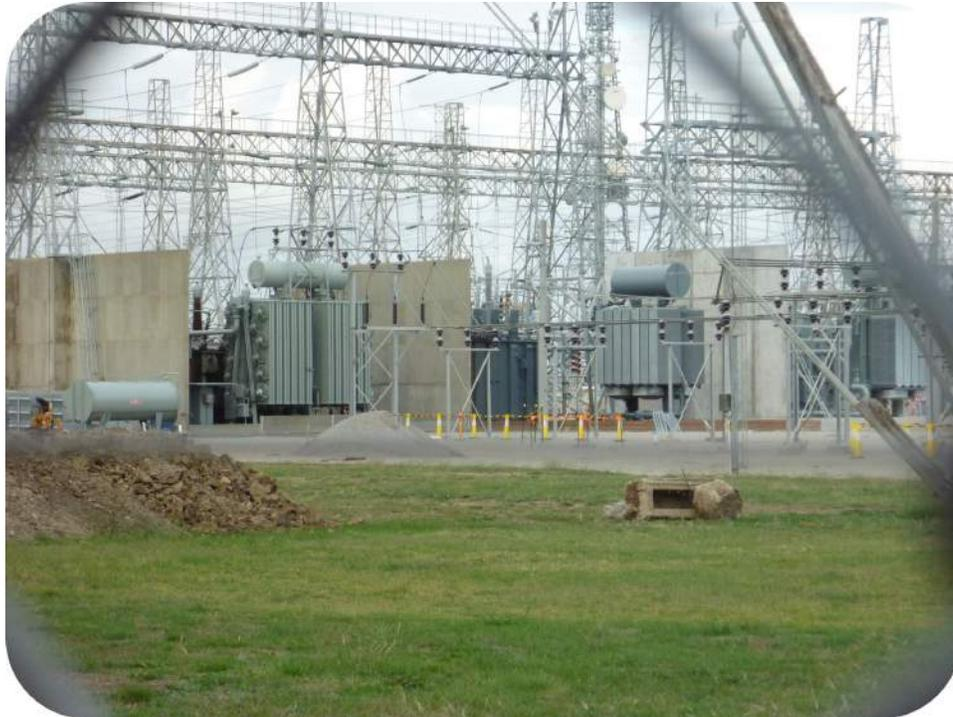
Part of the electrical grid, an electrical transmission sub-station receives extremely high current levels, then passes the electrical energy on to as many as 200,000 homes. Approximately 5000 megawatt-hours of energy passes through this particular substation each year.
