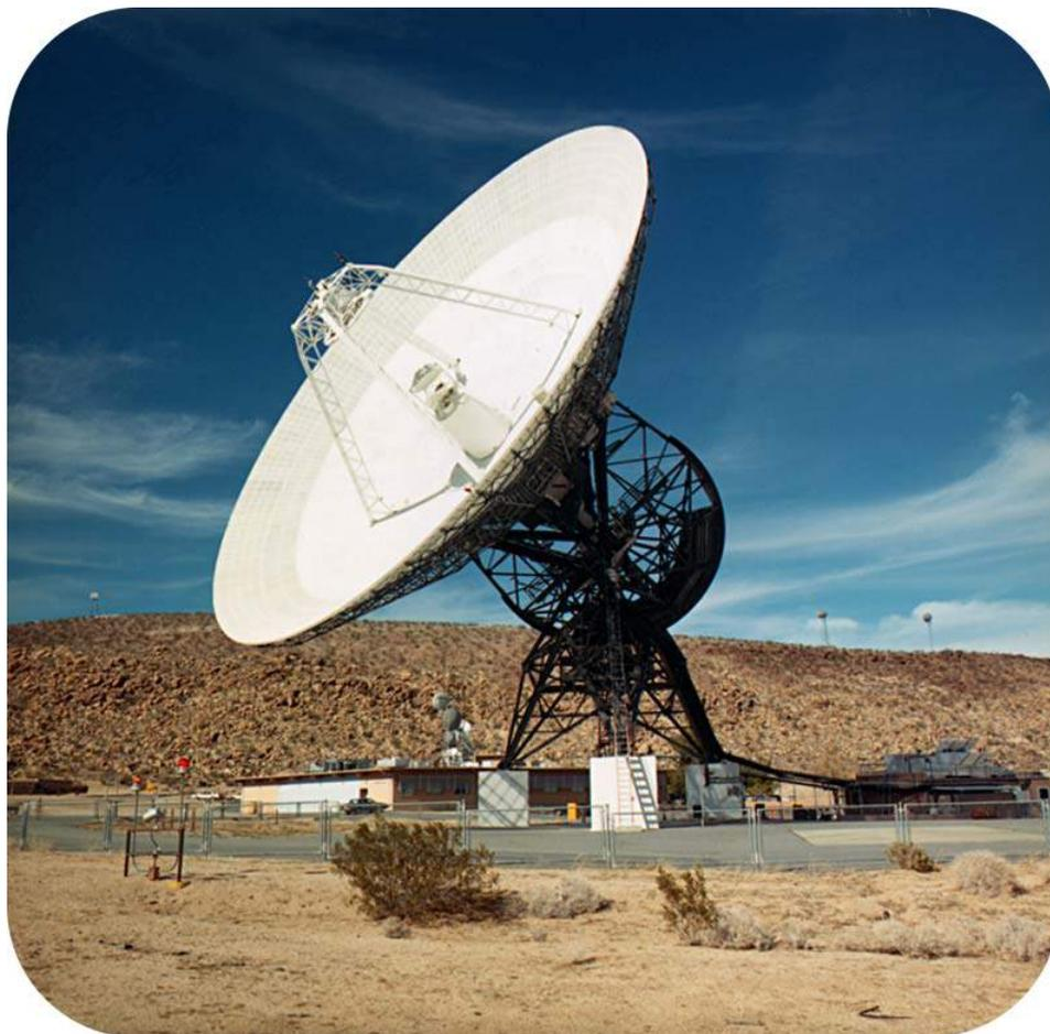
This is one of several large parabolic antennas at the Goldstone complex of the worldwide Deep Space Network that Jet Propulsion Laboratory manages for NASA. It spans 112 feet from rim to rim and stands nine stories tall. NASA used it for years to communicate with ships and devices in solar system exploration missions such as the Mariner, Voyager, and Galileo. When newer antennas replaced this antenna in communications use, it was converted to a radio telescope.
